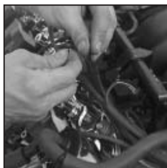
Wire tie the installed wires neatly
