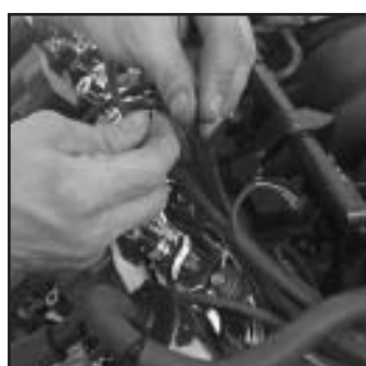
Wire tie the installed wires neatly
